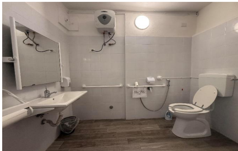
29 bathroom equipped with accessible sanitary facilities
